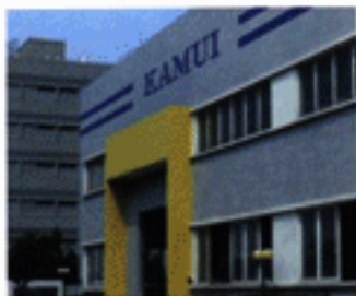
The shop for Air cooled cooler
