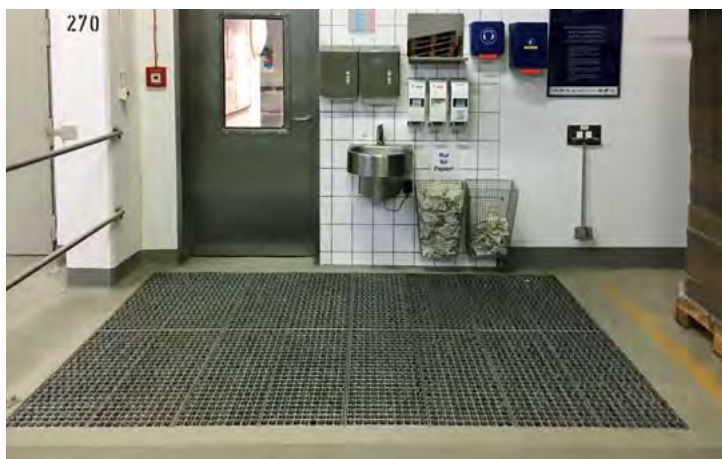
ProfilGate® go in front of the production-area entrance
