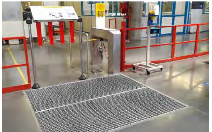
Cleaning of soles and rollers by ProfilGate® st55 go in front of the ESD-area
