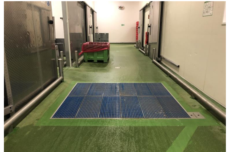
Picture: Hygiene sluice in Meat Processing factory
